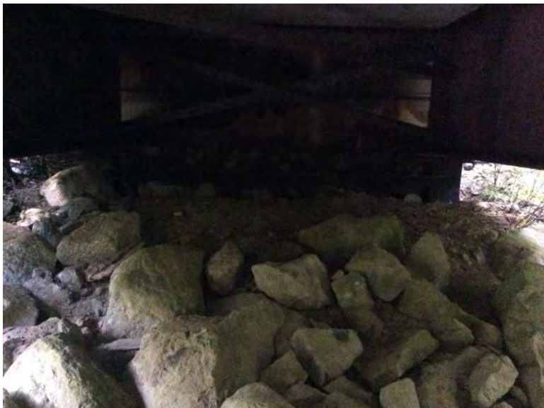
Left Bank Abutment when facing downstream
