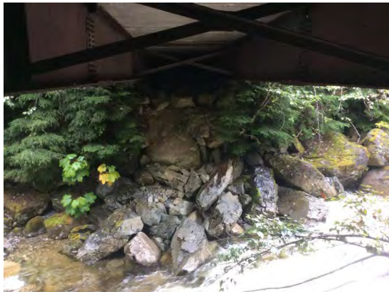
Right Bank Abutment when facing downstream
